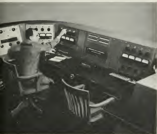
key point in world-wide broadcast service is this control console at RCA Communications in New York.
